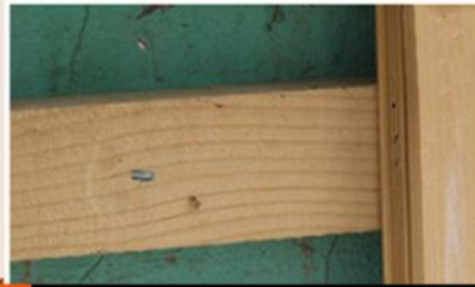
02 Secure the wooden keel with steel nails
