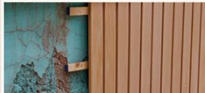
01 Clean the wall before installation
