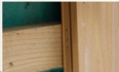
03 Tilt the air gun nail into the socket
